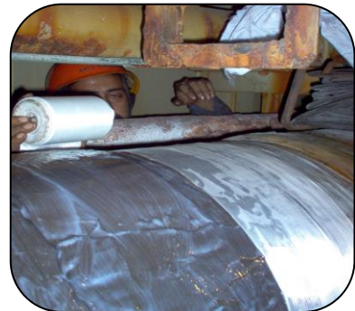
Badly corroded ballast pipe manually prepared and filled using 302 Epoxy Repair Cement, 30mtr length of pipe then encapsulated using 301 Epoxy Resin and Hardener and Glass Tape
