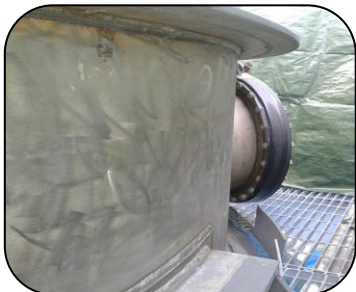
95°C evaporator surface filled using 107 Metal Repair Paste XL prior to the application of 561 Thermal Barrier
