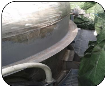
95°C evaporator surface filled using 107 Metal Repair Paste XL prior to the application of 561 Thermal Barrier
