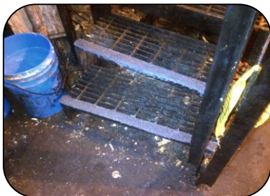
Oil refinery steel steps degreased and coated with 104 Metal Repair Fluid XF and Aluminium Oxide aggregate. No sparks were allowed in the repair area, the material bonded to the substrate even with oil contamination on the surface.
