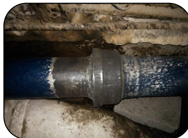
Oil refinery pipe line socket joints manually prepared then coated and wrapped using 104 Metal Repair Fluid XF.
