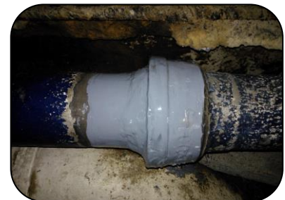
Oil refinery pipe line socket joints manually prepared then coated and wrapped using 104 Metal Repair Fluid XF.
