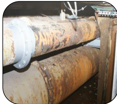
Badly corroded sea water lines encapsulated using 301 Epoxy Resin and hardener and 3 x wraps of Glass Tape
