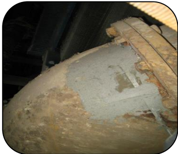
Eroded gas main repaired using 301 Epoxy Resin and Hardener and 3 x wraps of Glass Tape
