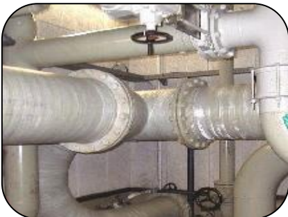
Main fire water lines encapsulated using 301 Epoxy Resin and Hardener and 3 x wraps of Glass Tape
