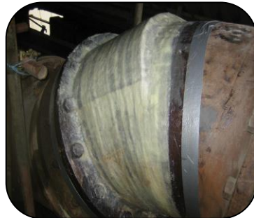
Eroded gas main repaired using 301 Epoxy Resin and Hardener and 3 x wraps of Glass Tape
