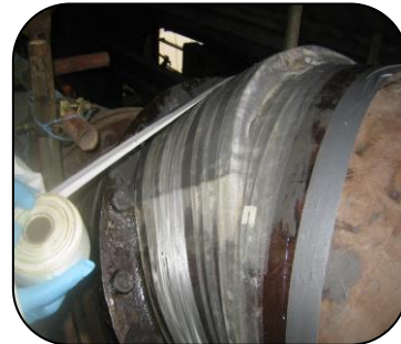
Eroded gas main repaired using 301 Epoxy Resin and Hardener and 3 x wraps of Glass Tape
