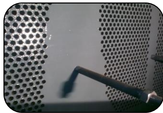
Condenser tube sheet resurfaced
