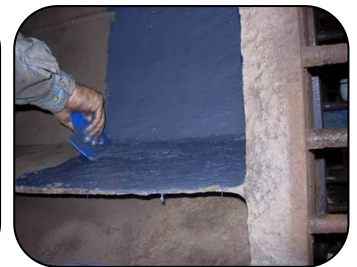
Process vessel surfaces badly corroded from chemical attack rebuilt using 201 Ceramic Repair Paste
