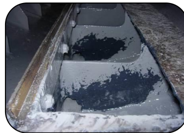
Process vessel surfaces badly corroded from chemical attack rebuilt using 201 Ceramic Repair Paste
