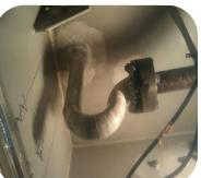
Accommodation area waste water pipes were leaking at the welded joints. Over 60 bends and joins wrapped using 301 standard resin and hardener and glass tape
