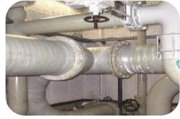
Sea water lines in an engine room encapsulated using 301 Standard resin and hardener and 100mm wide glass tape. Three wraps of this system onto manually prepared surfaces will resist 75-100psi pressure
